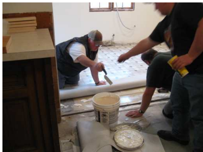
Frank, Ken and Zack laying the new linoleum.
