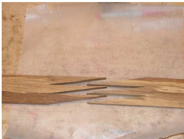
Cut out Z-Splice ready to be glued up.
