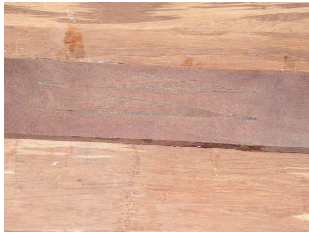
Glued up Z-Splice, ready for backing.
